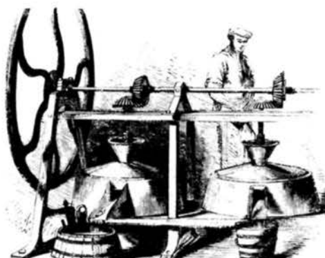
315. COLOUR-GRINDING MACHINE.
